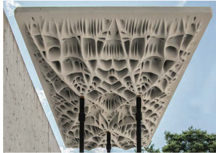
Prototype "A" slab, 80% mass reduction Credit: Andrei Jipa et al.
